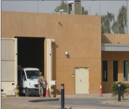
Guard inspecting entering vehicle
